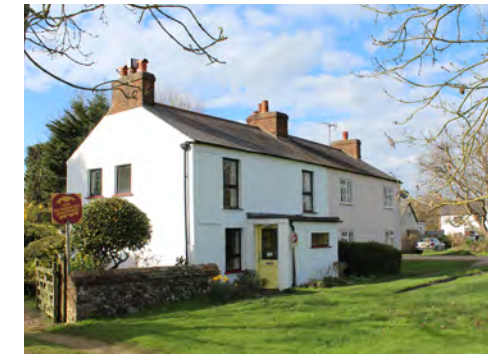
Figure 29 South and Smiths Cottage
